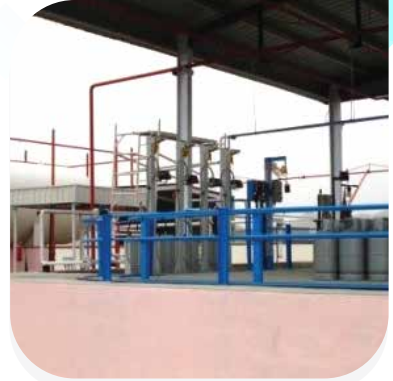
Setting up LPG Bottling Plant
